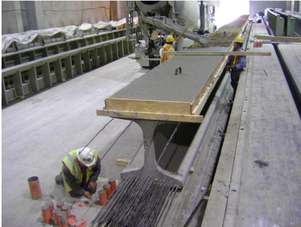
Figure 3.25 NU1100 Deck Pouring
