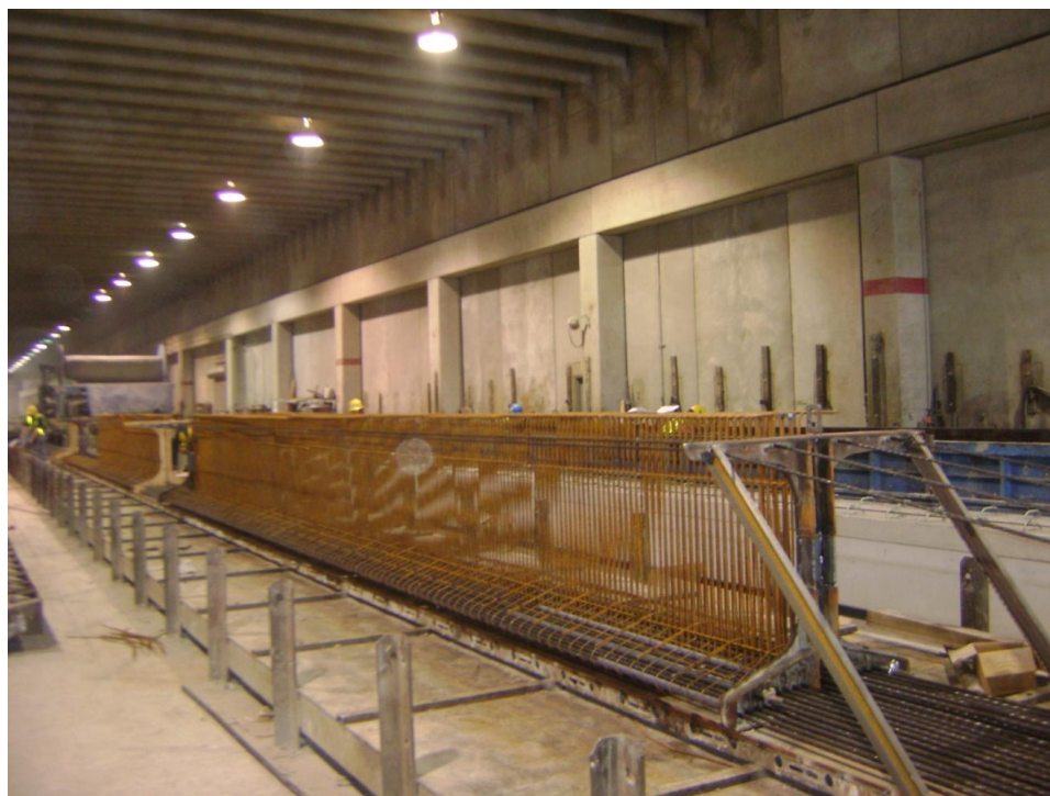
Figure 3.20 NU1100 Reinforcement
