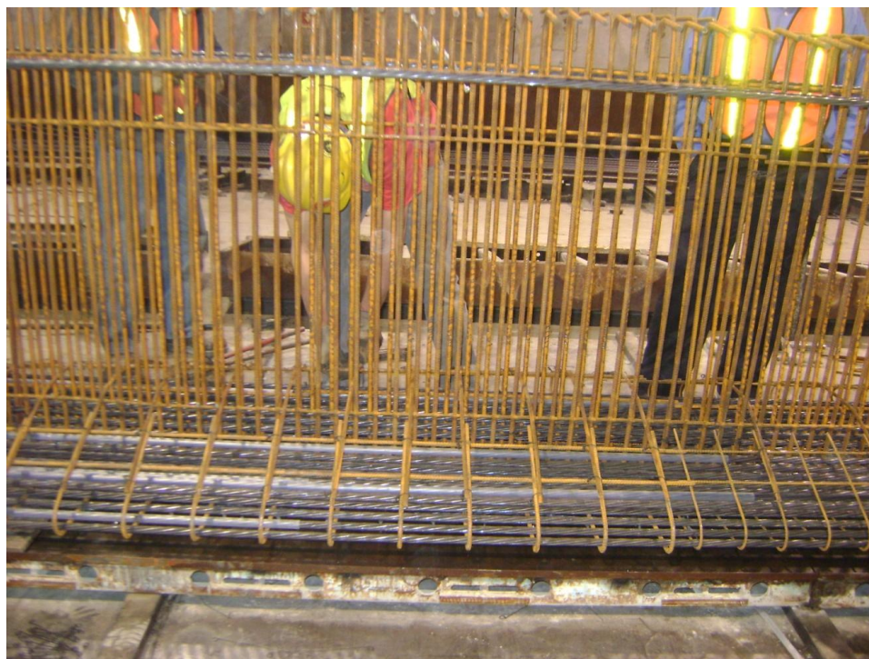
Figure 3.21 NU1100 Confinement Reinforcement
