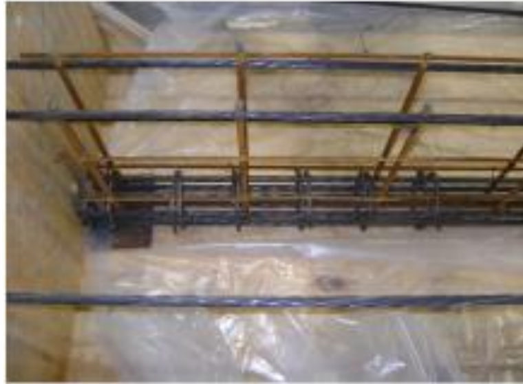
Figure 3.6 T24 End Confinement
